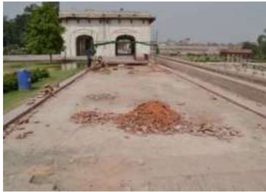
Figure 22: Walkways towards Aiwan (Summer Pavilion) during conservation work
