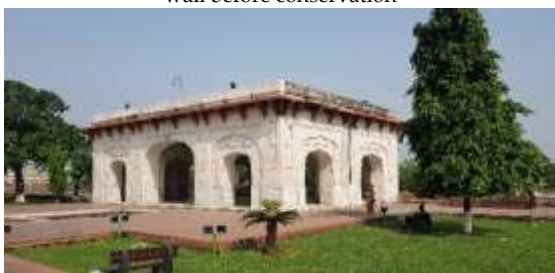
Figure 31: Glaze plaster work of certain parts of parapet wall after conservation (Source: Author)
