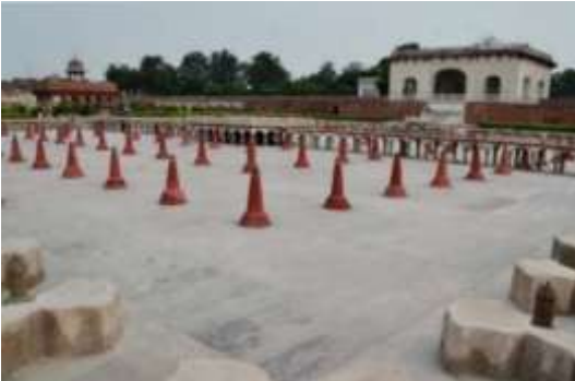
Figure 53: Full view of fountains tank after rehabilitation
