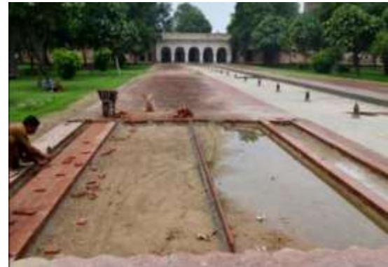
Figure 26: Left side walkways towards Khuwabgah (Residence of Princess) during conservation work
