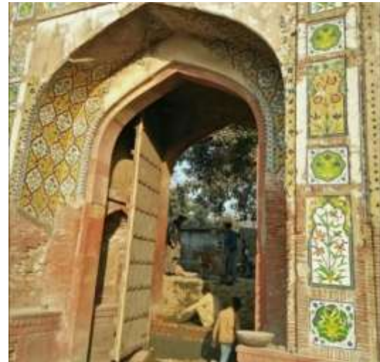
Figure 66: Conservation And preservation work of gates in process.
