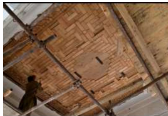
Figure 32: Tarseem-Bandi During Conservation and Preservation of Summer Palace/Aiwan
