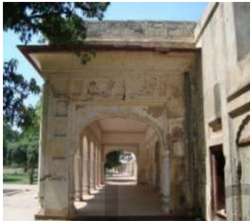
Figure 35: Before Conservation of Pavilion integral part of Naqqar Khana Complex
