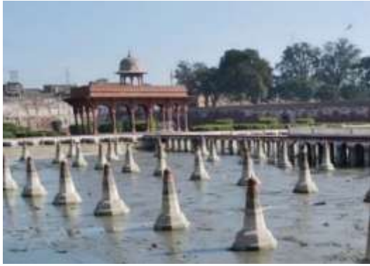
Figure 52: Full view of fountains tank before rehabilitation
