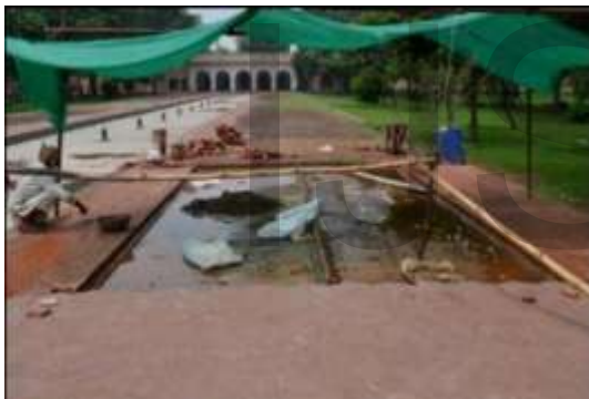
Figure 24: Right side walkways towards Khuwabgah (Residence of Princess) During Conservation work
