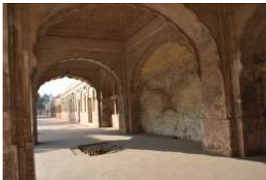
Figure 43: Fountain's condition before restoration at interior of north gate, original openings at right have been bricked over
