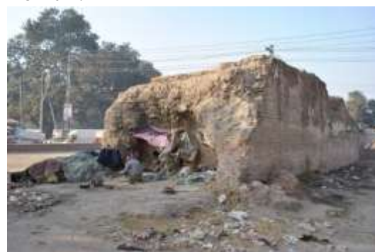
Figure 56: Demolished remains of Hydraulic tank when the G.T road was widened to its present size in 1990s.
