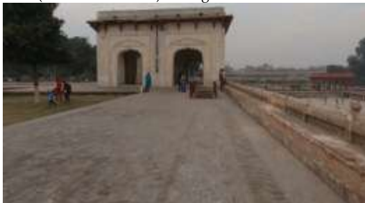
Figure 23: Walkways condition towards Aiwan after conservation work
