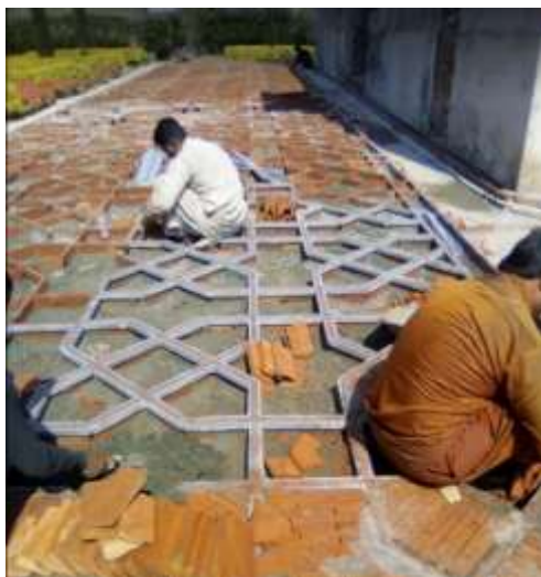
Figure 15: During Restoration work at Gulabi Gate
