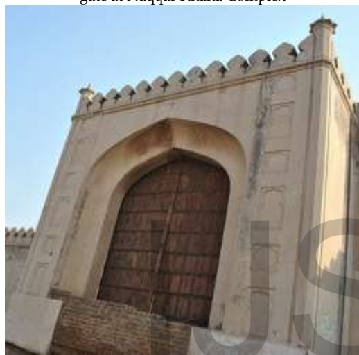
Figure 42: Restoration of wooden north gate at Naqqar Khana Complex
