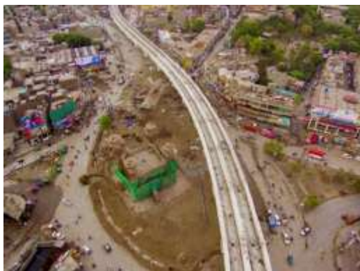
Figure 12: Netting/Sheeting and Bracing During Orange Line Metro Train (OLMT) project
