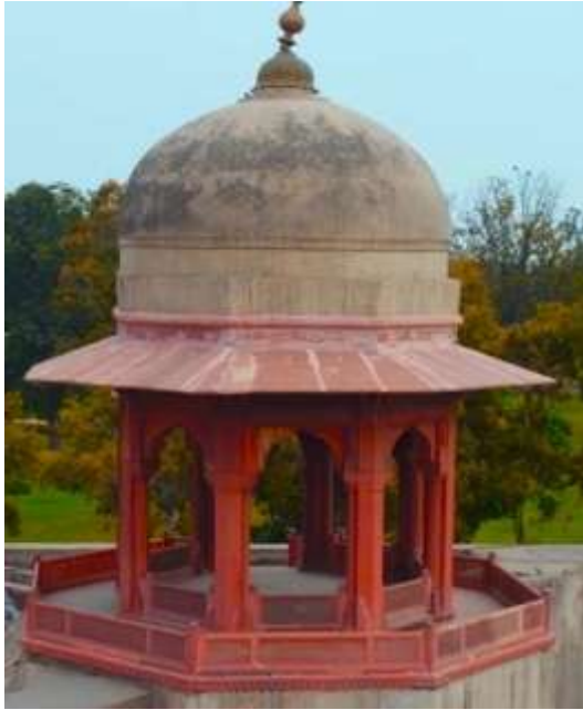
Figure 63: Closer view After Rehabilitation of Burj at Shalimar gardens.
