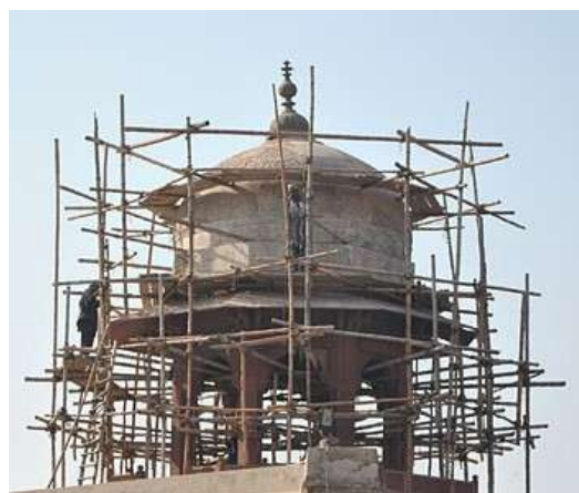
Figure 62: Closer view During Rehabilitation work of Burj at Shalimar gardens.
