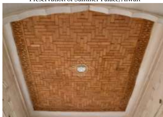
Figure 33: Completion of Tarseem-Bandi of Ceiling at Aiwan
