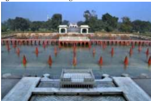
Figure 55: View from King's throne after rehabilitation
