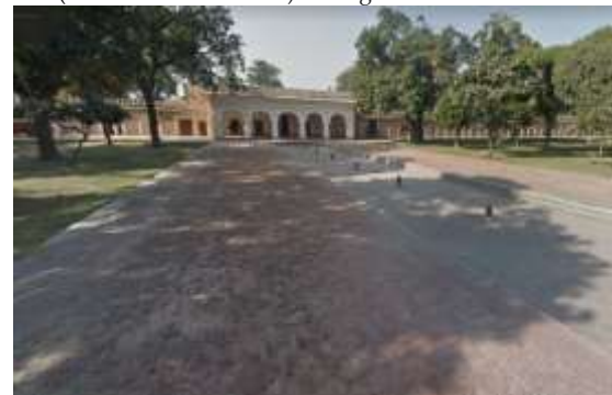
Figure 27: Left side walkways towards Khuwabgah (Residence of Princess) after conservation work
